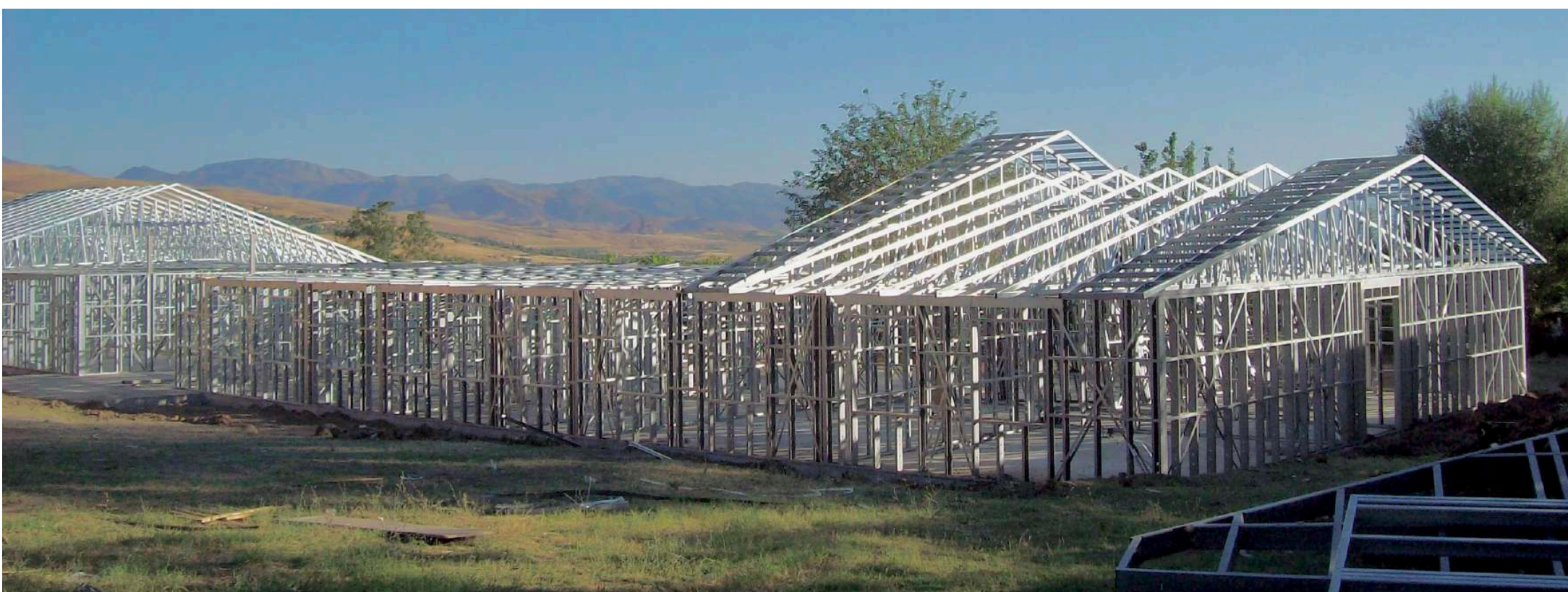
APEC - Besiktas Elementary School, Elazig Turkey
