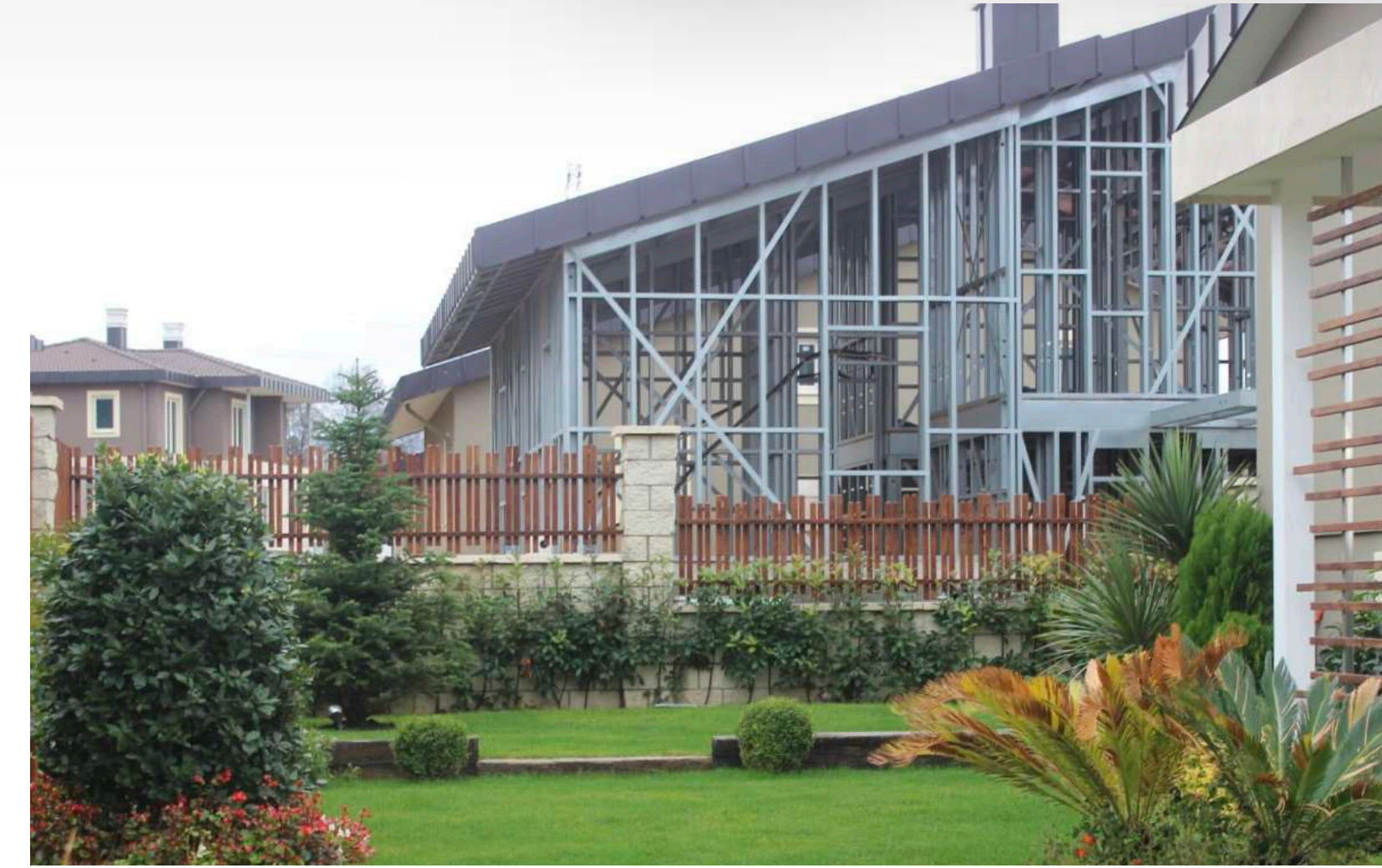
Sakura Park Yalova, Construction Process
