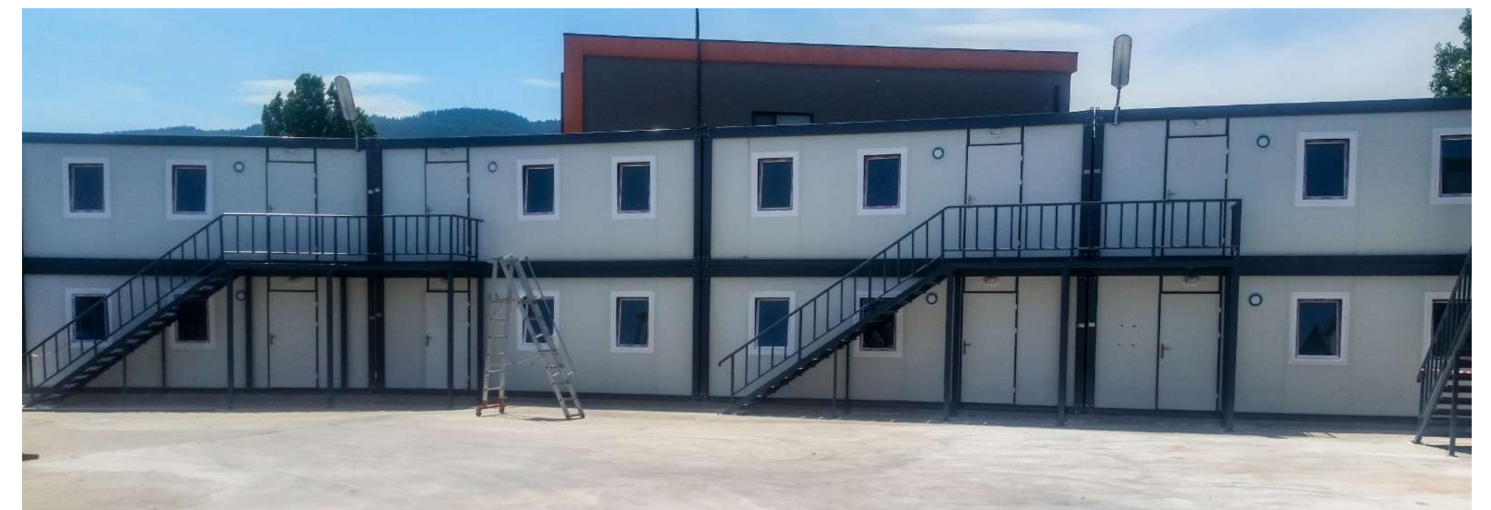
Container Labor Camp, Finland
